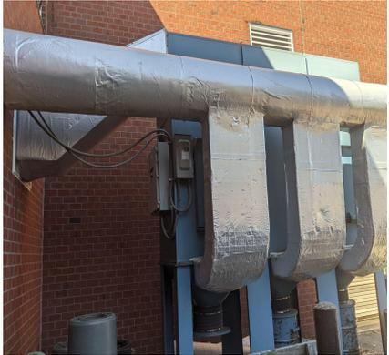
A photograph showing a large, industrial dust collector system with silver ductwork and blue structural supports, situated outdoors against a brick wall. |
