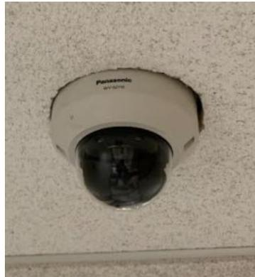
MHS - Current camera system is outdated and does not support the needs of the school. Cameras need to be replaced and current server is not adequate.
